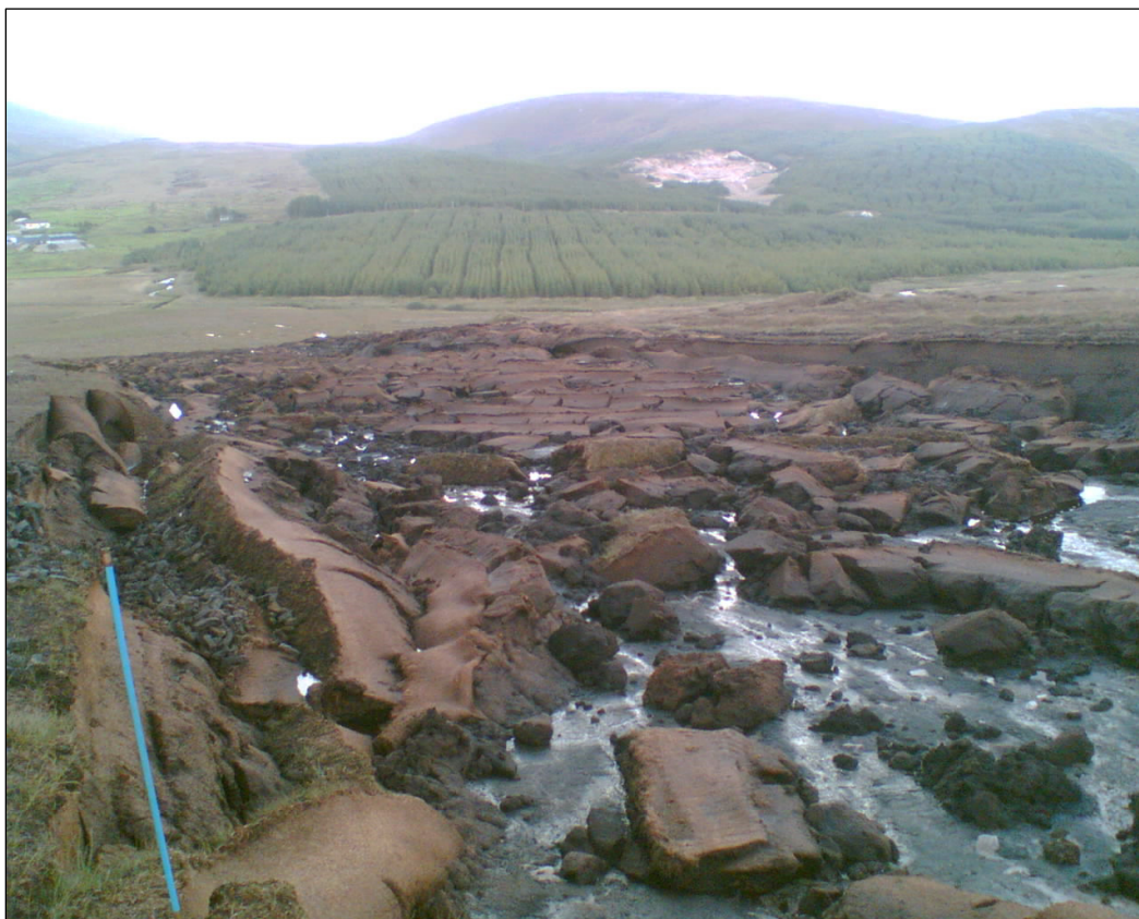
Figure 4.4: Peat failure, Glencolumcille, Co. Donegal showing a peat failure within a machine cut area of peat. (Photo courtesy of Dr Paul Jennings)
