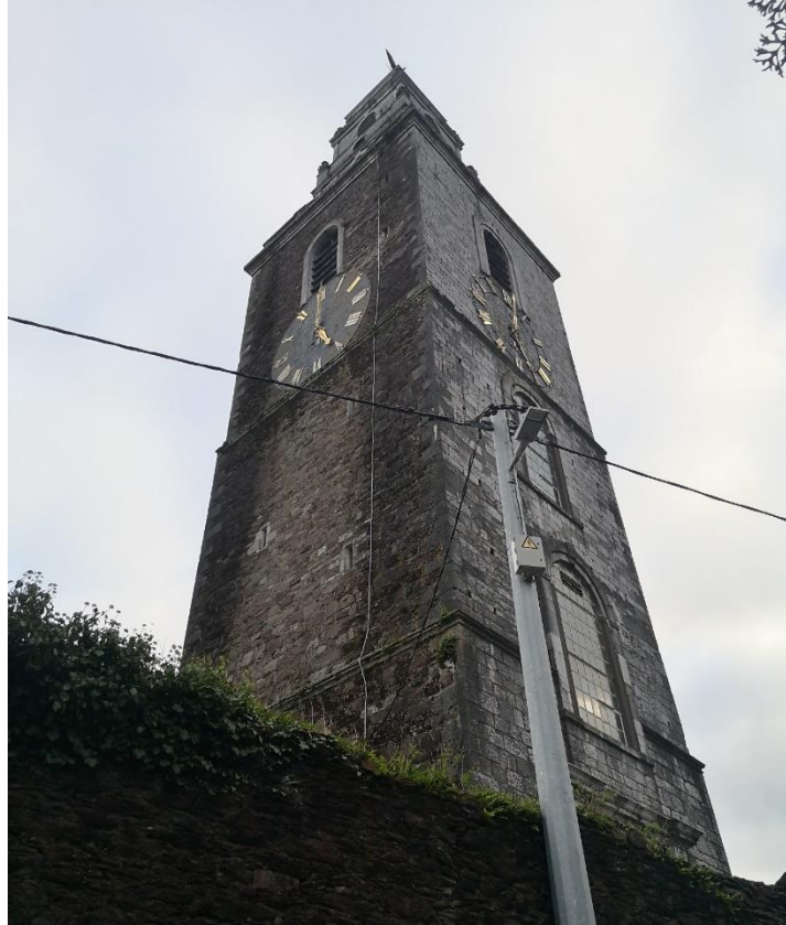
The north side (left) of the tower, made of red sandstone, and the west side (right), built from limestone.
