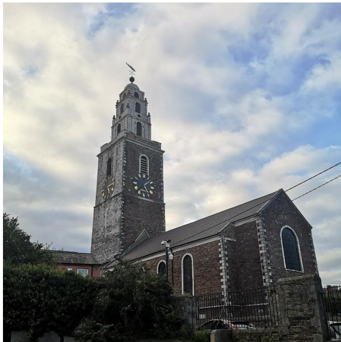
The east side (right) of the tower, made of red sandstone, and the south side (left), built from limestone. The rest of the church body is sandstone, with limestone finishings around windows and the corners of the building.
