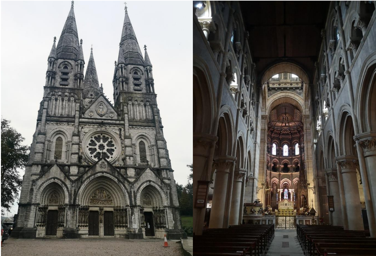
Left: external façade of St Fin Barre's Cathedral, primarily of Beaumont Dove Limestone – the statues around the doors are from Ballinasloe Limestone. Right: internal dressings, with marble of unknown provenance in the apse, and Bath Stone pillars.
