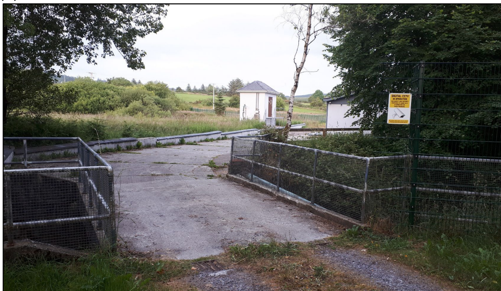
Springs in marshy area to north (left) of pumping station complex.
