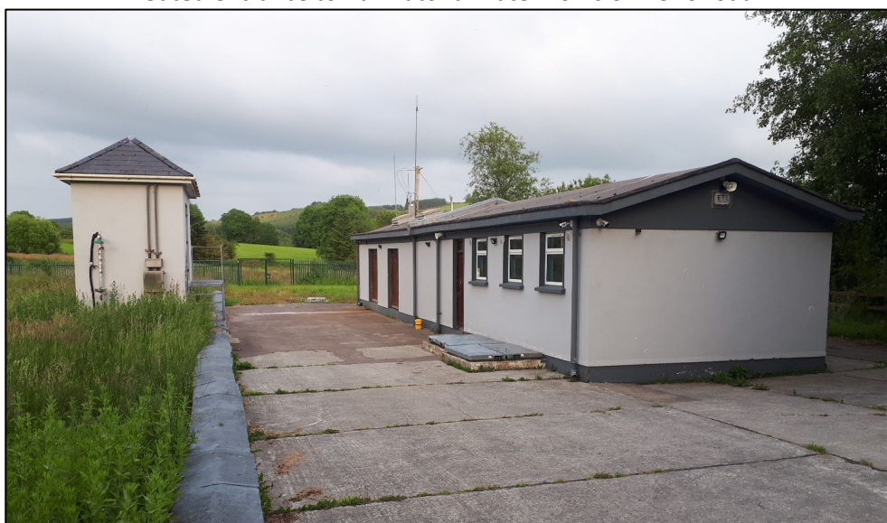
Ballinatonna Waterworks Pumping Station.
