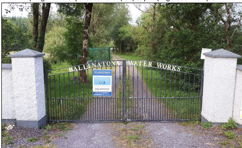
Gated entrance to Ballinatonna Waterworks on R576 road.
