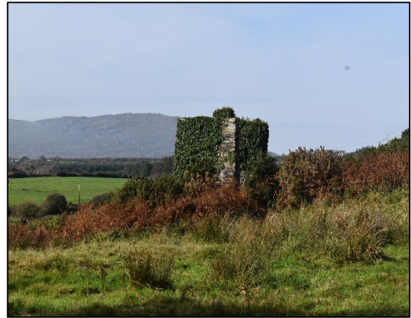
Pillar-like mine buildings at southwestern end of site, showing overgrowth by vegetation (mainly ivy) since 2007.
