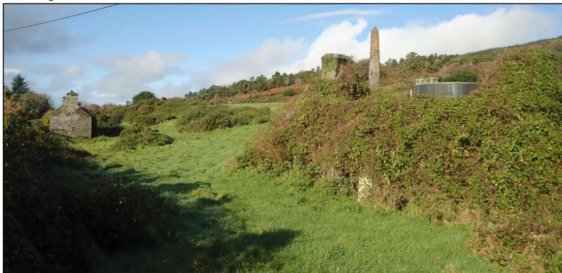
The chimney and old quarry buildings at Benduff Slate Quarry, viewed from the southeast.
