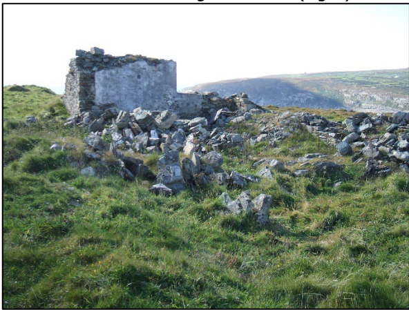
Remains of engine house at Brow Head Mine.
