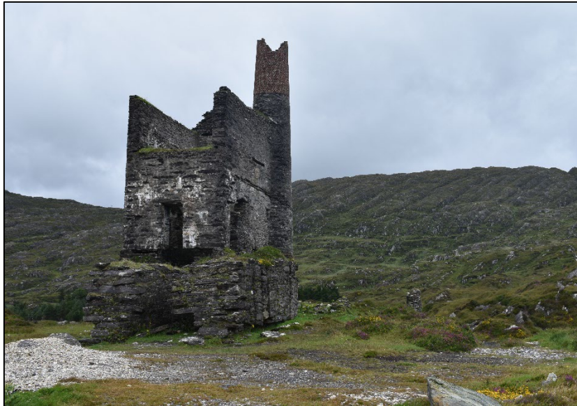
Coom engine house, view from south. The bob wall is visible and overlooks the engine shaft (out of shot, to the left), known as Bewley's Shaft.
