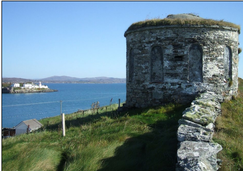
Powder house (magazine) on south side of mine site, view to east (Photo taken 2007).
