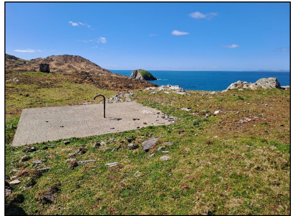
Concrete capping on mine-shaft.
