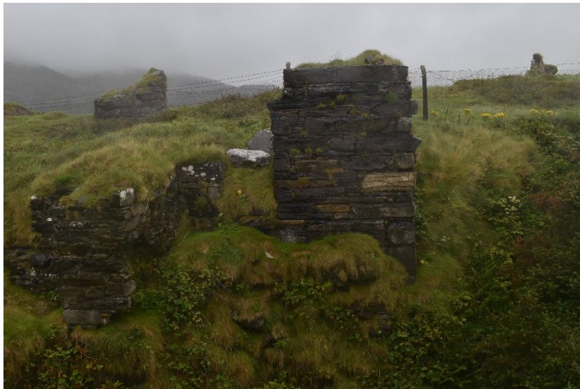
Remains of engine house at Dooneen Mine in fenced area east of road, with base of chimney in background (left).
