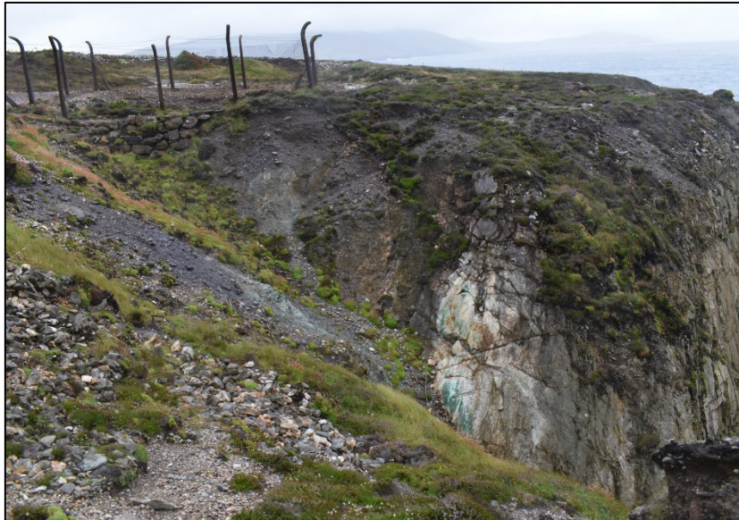
Malachite staining on exposed vein extending out from cliff face. The fenced Footway shaft is visible to the left.
