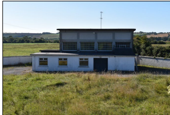
Dower Spring plant building.
