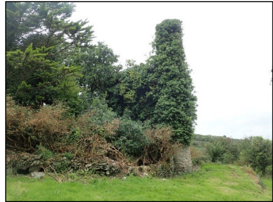
The chimney and engine house on the site.
