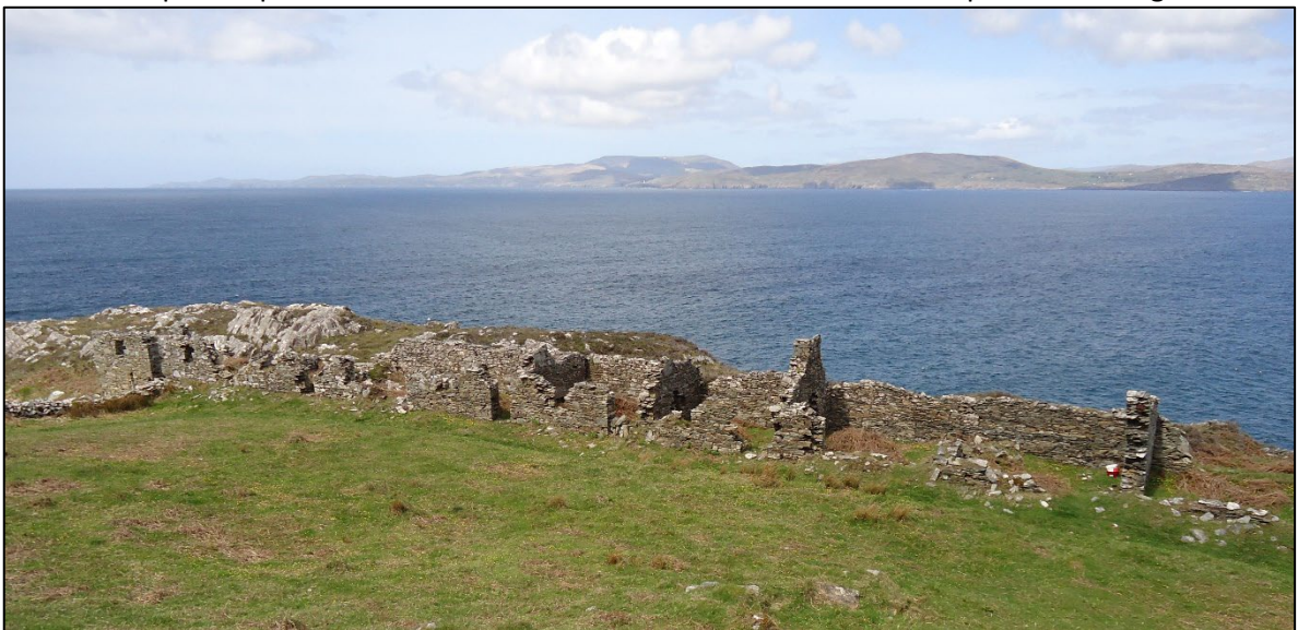
Miner's cottages to the west of the mine site. Slieve Mickish on Beara peninsula visible to north across Bantry Bay. Allihies Copper Mines were situated west of Slieve Mickish.
