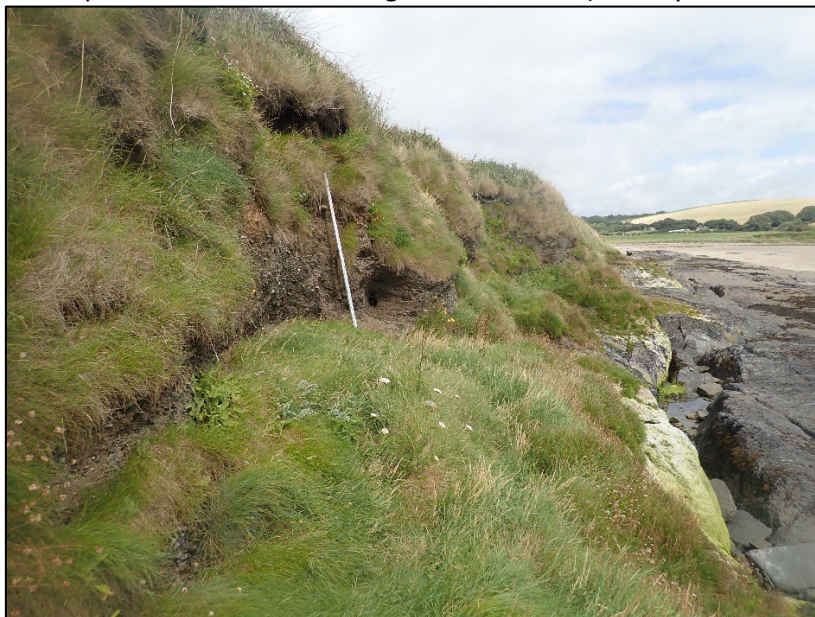
The diamicton overlying the raised beach sands and gravels atop the rock platform along the western side of Howe's Strand. Staff here is 2 m long.
