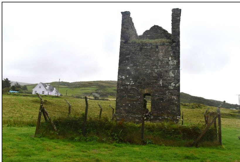
Puxley's engine house, view from west of the bob wall. The fenced engine shaft is in foreground.
