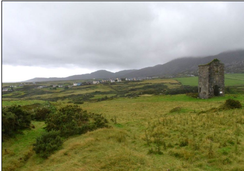
General view of Kealogue Mine (North), view from the southeast.
