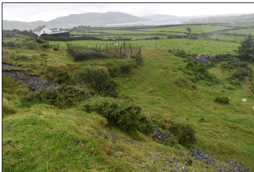
View westwards from beside the engine shaft along steep bank of mine waste, with a second fenced shaft visible 40 m distant.
