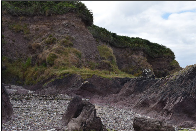
Knockadoon Head, south of pier - cliff of till resting on wave-cut platform.
