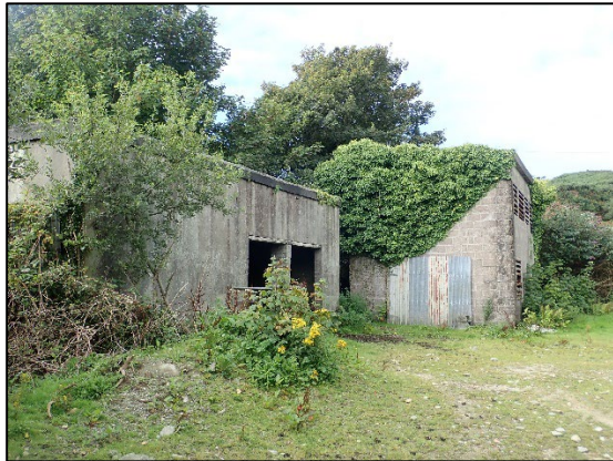
Some of the mine buildings on the pit floor.
