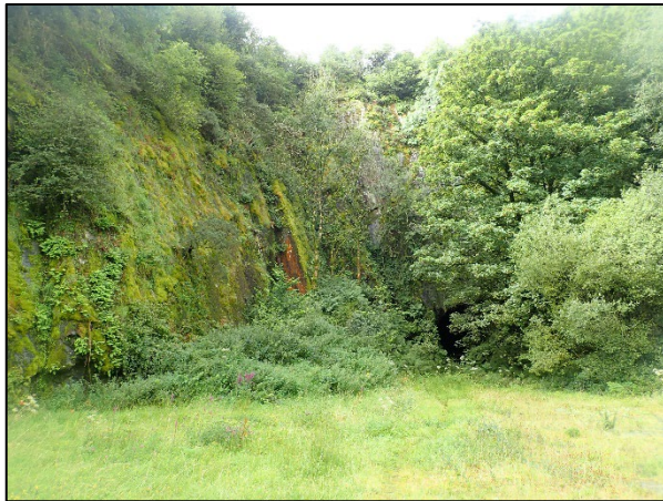
The entrance to the underground galleries, partially-obscured by scrub.
