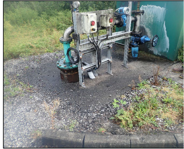
Water supply borehole from the eastern end of the site.
