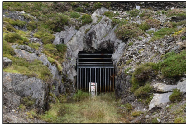
Entrance to Main Adit, viewed from south.
