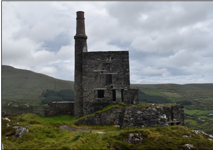
Man Engine House, view towards south.
