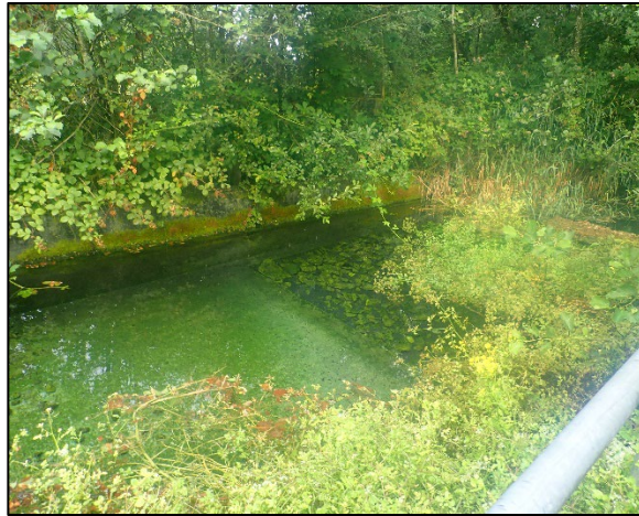
The sump between the spring and the weir.
