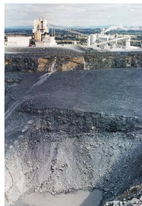
The lime kilns and quarry plant.
