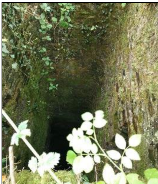
Interior wall of uncapped shaft showing rounded corners.
