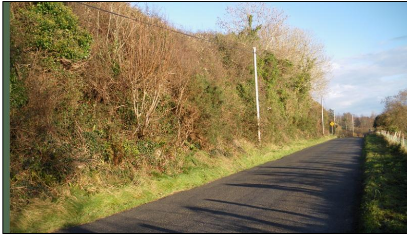
Western road cutting, heavily overgrown (view to east).
