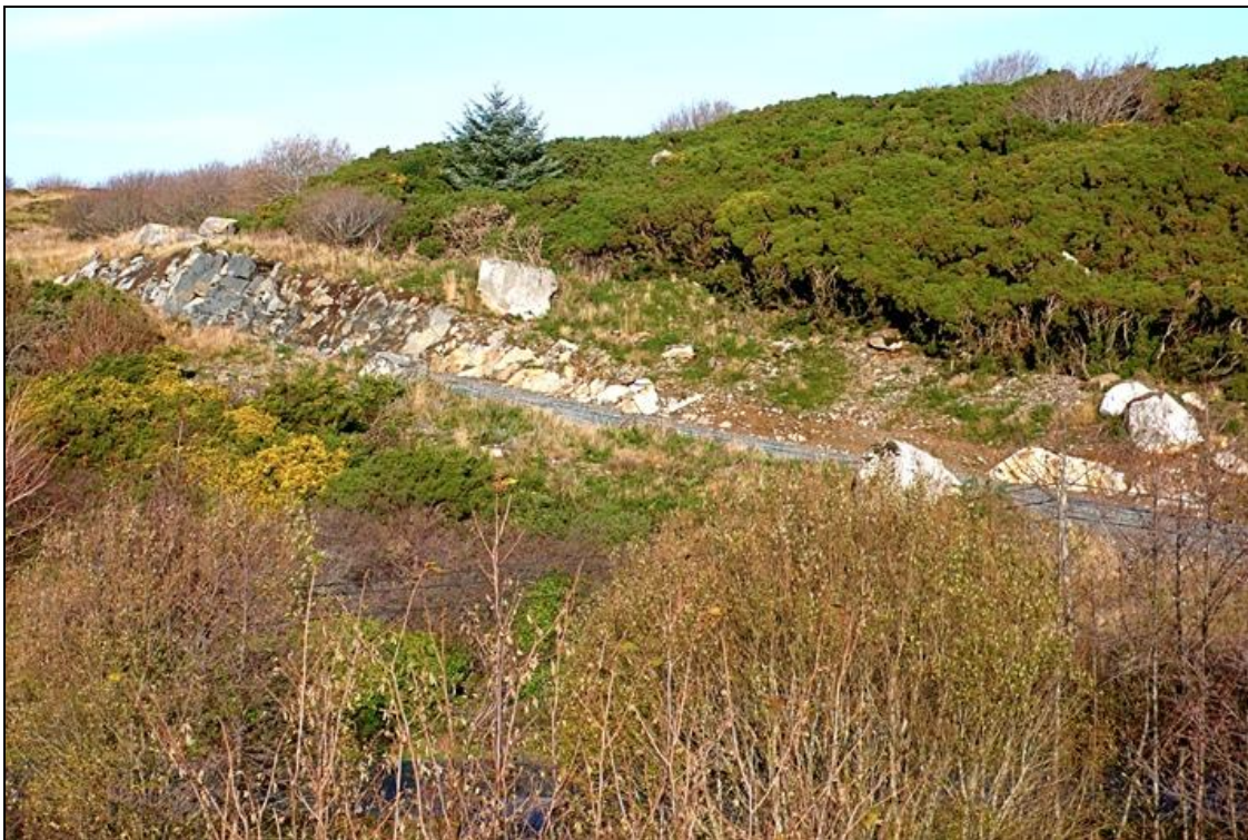
New roadway through contact metamorphic aureole; metadolerite sill visible on left (grey colour).
