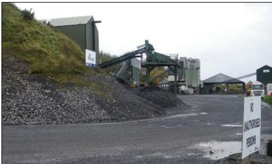
Western quarry, aggregate processing plant.
