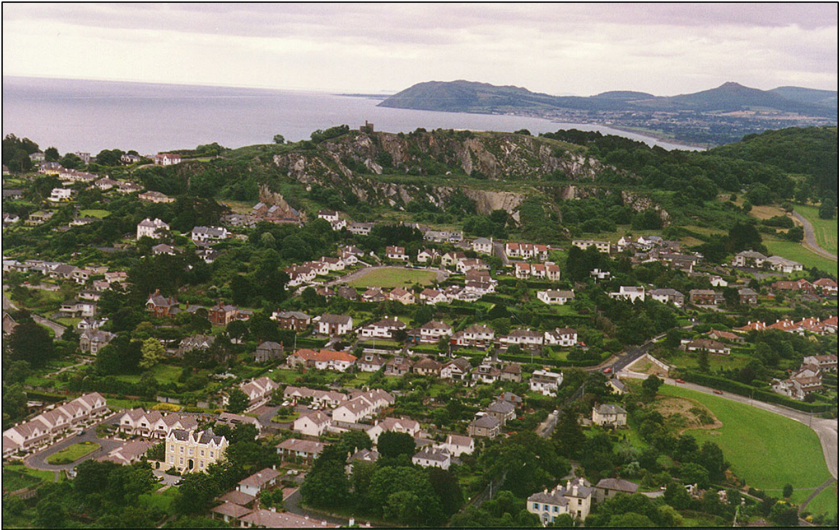
An aerial photograph of the quarry, with two levels apparent and the central inclined ramp that supported the metals – the rails of a rail system for transporting rock to Dun Laoghaire.
