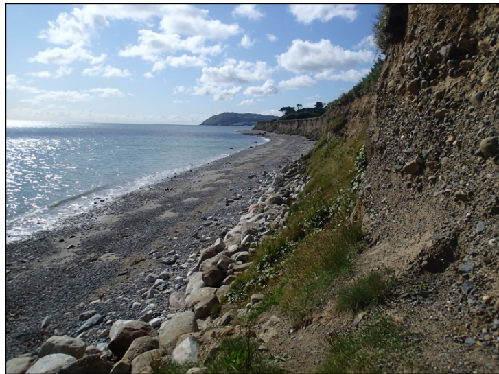
Left: Gravel beds resting on top of stiff, muddy glacial till sediment in the coastal section at Shanganagh Townland. Right: Looking south along the section from Corbawn Lane, with the huge recently installed 'rock armour' boulders set as coastal protection clearly seen.
