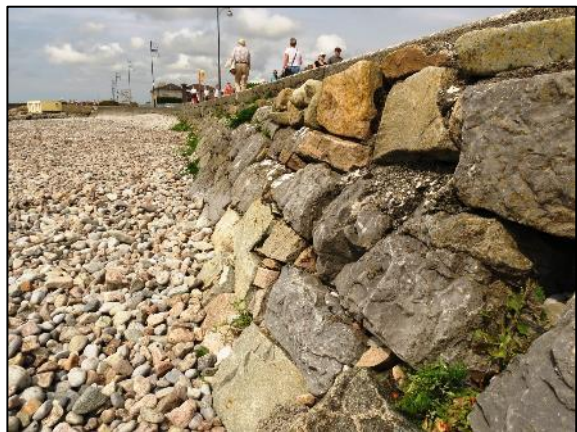
Granite, limestone and metagabbro blocks in seawall below promenade opposite Galway Bay Hotel.
