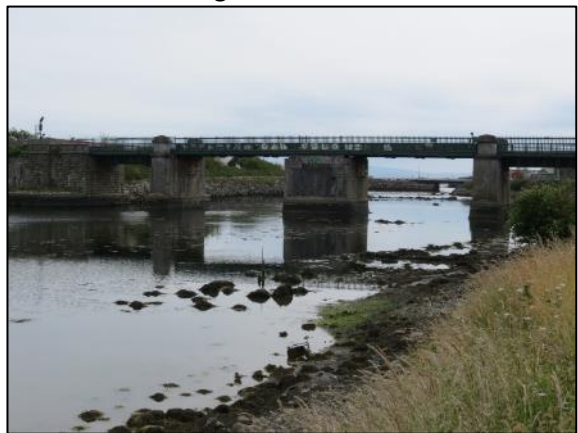
Channel to Galway Bay beneath railway bridge.
