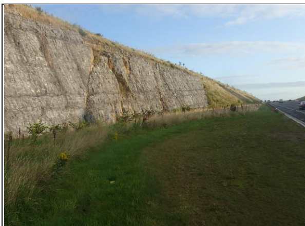
Groundwater seepage beneath epikarst layer, and potential karstified bedrock cavities.
