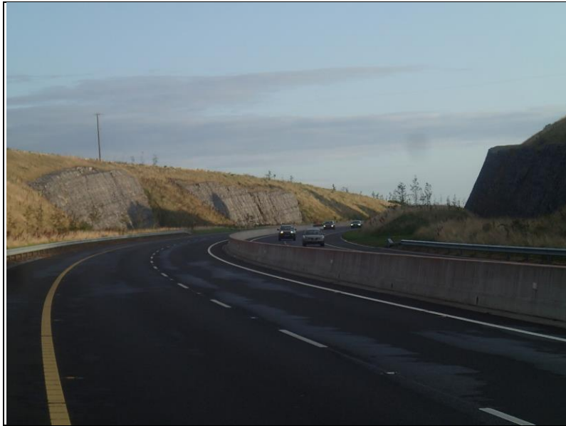
View north along the Ballybanagher road cut along the M17.
