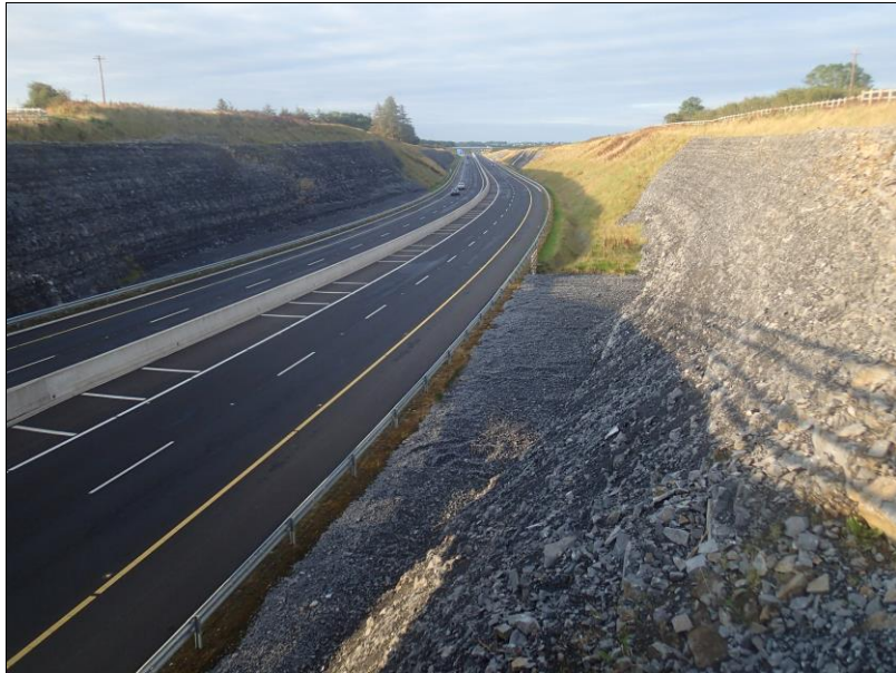
View south along the Caherateemore road cut along the M17.
