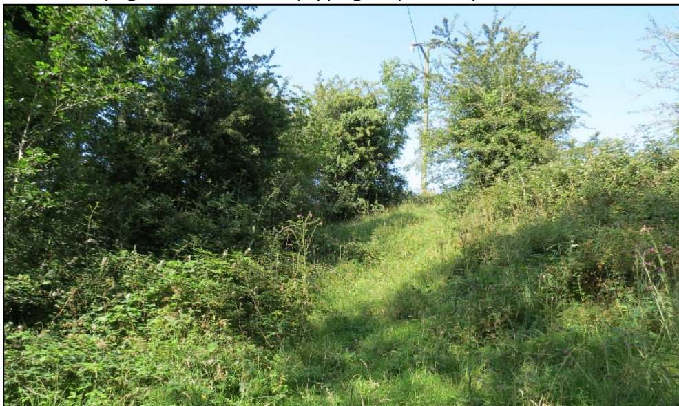
Steep slope from streambed (NW bank) up to surrounding pasture-land level. Slope indicates depth at which stream has cut into thick till deposits.
