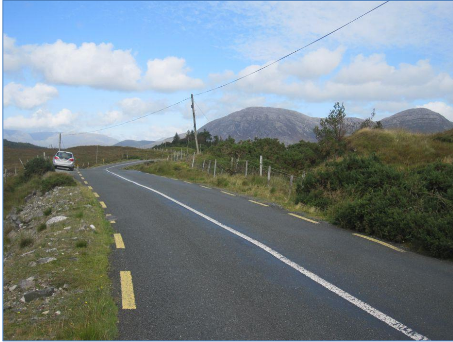
The roadside excavation at Cloonnacartan.
