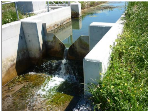
The weir for measuring spring overflows at Gortgarrow, July 2018.
