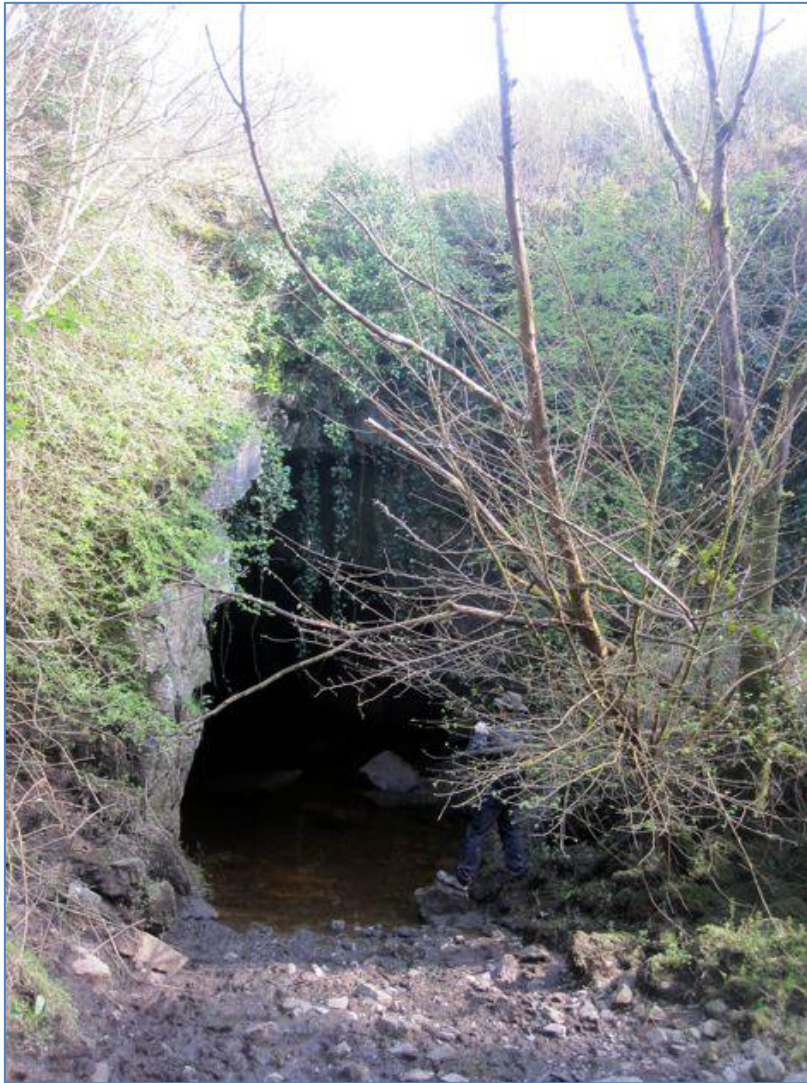
View of Pollaloughabo entrance showing the permanent intersection with the water table.
