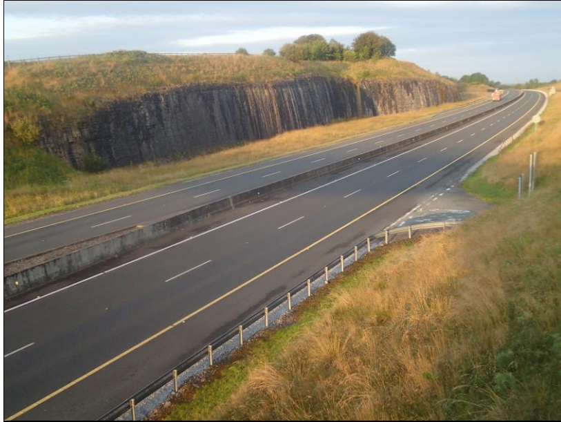
View west along the Rahally road cut along the M6.
