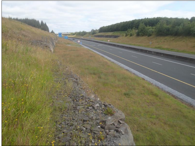
View east along the Toormore road cut along the M6.
