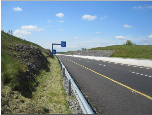
General view at north end, looking south.
