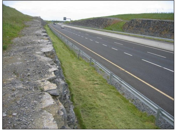
General view looking north.
