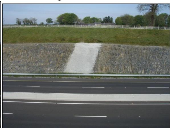
Concrete patch reinforcing weak ground.
