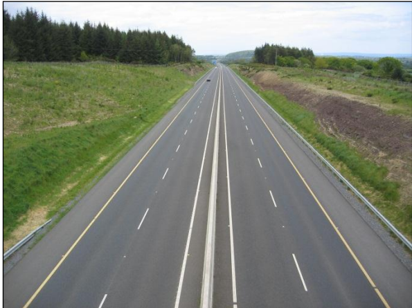
View of cuttings from the over bridge.
