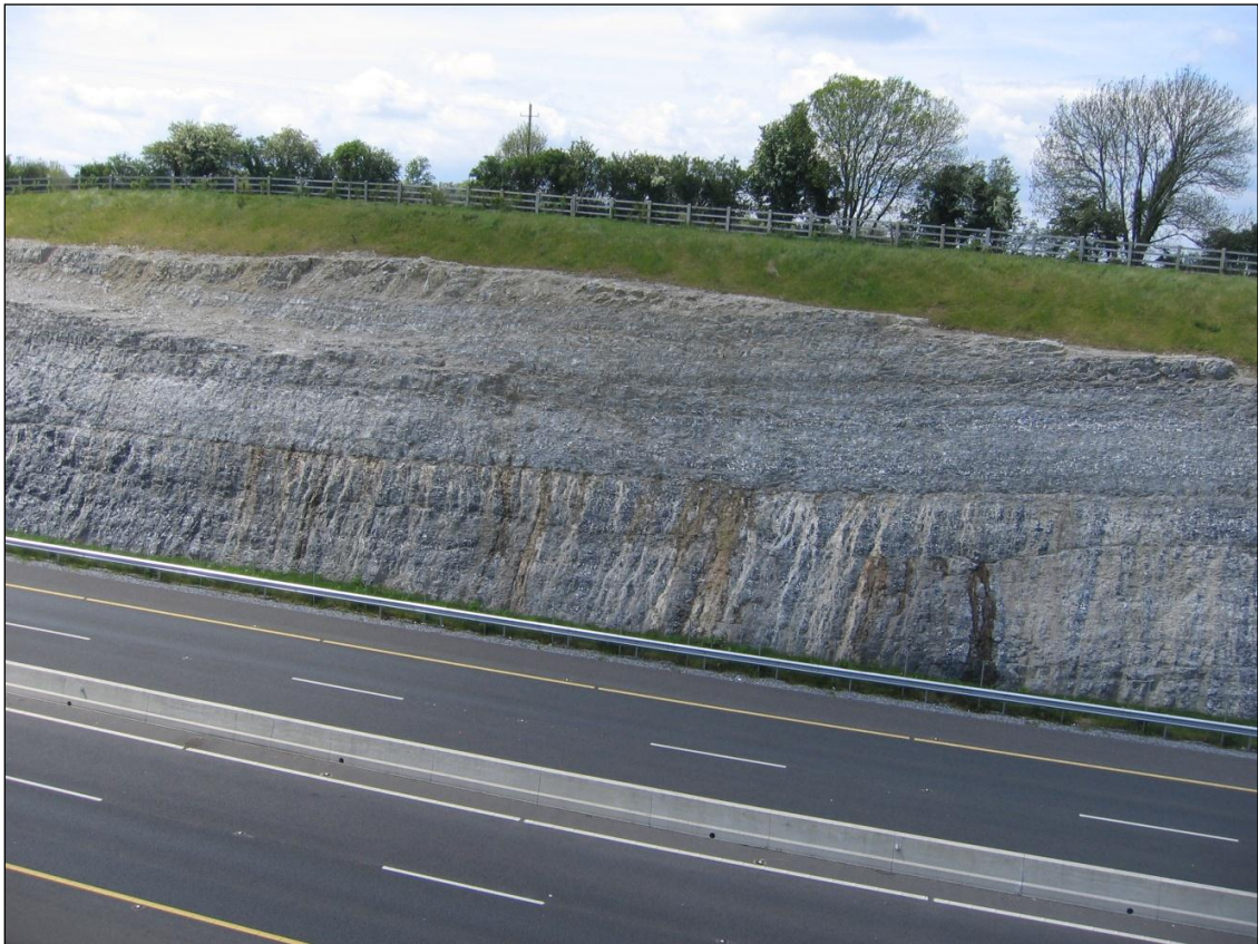
A view of the west side of the cutting clearly showing the changes in bedding half way up the face and the lime stains of water flows from the bedding plane of the junction.
