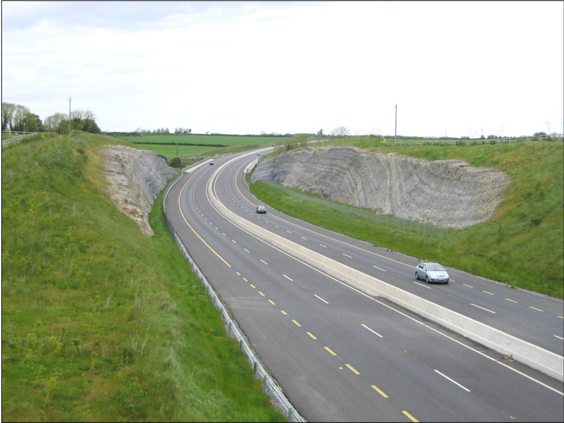
A view looking north of the King's River cutting with obvious folding on the right hand (east) side.
