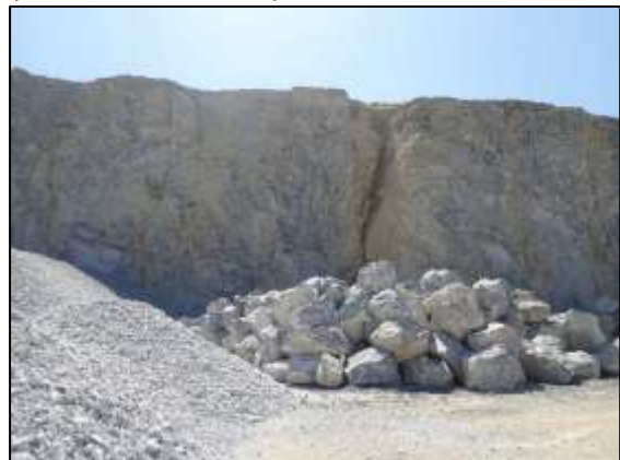
A narrow, deep, clay-filled, karstified fracture in the limestone.
