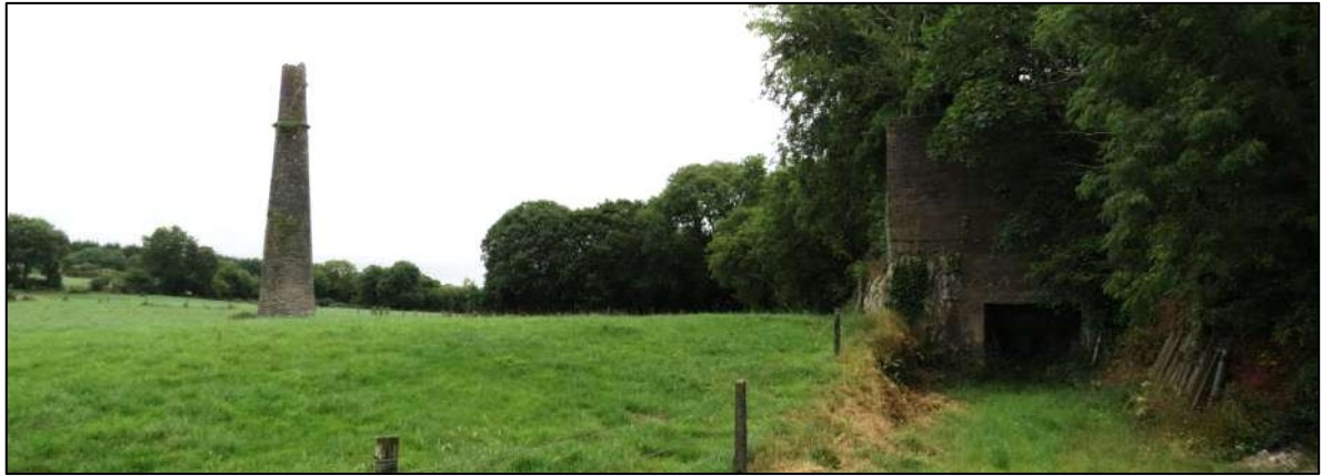
Site of Ardtully Mine. Chimney stack and lime kiln.
