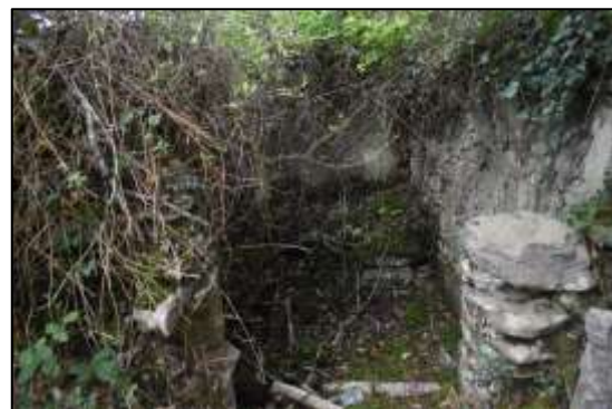
Old mine site east of Camillan Bay: ruined, presumably mine building, of unknown purpose, at western end of site. View of interior from east.
