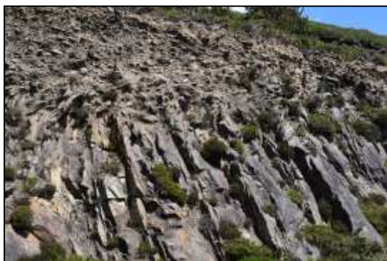
Road cutting at Red Cliff, east of the road bend, showing bending and extensive shattering and break-up of sandstone beds in contact with overlying glacial till in response to solifluction.
