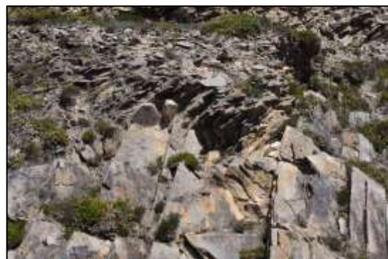
Road cutting at Red Cliff, close to lay-by east of the road bend, showing bending and extensive shattering and break-up of sandstone beds in contact with overlying glacial till in response to solifluction.
