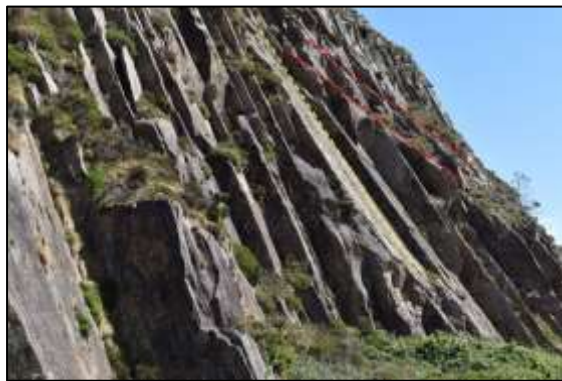
Close-up of Red Cliff road cutting at bend in road: steeply dipping beds (foresets) (dashed yellow line to illustrate), truncated by less steeply inclined erosional surfaces (dashed red lines).
