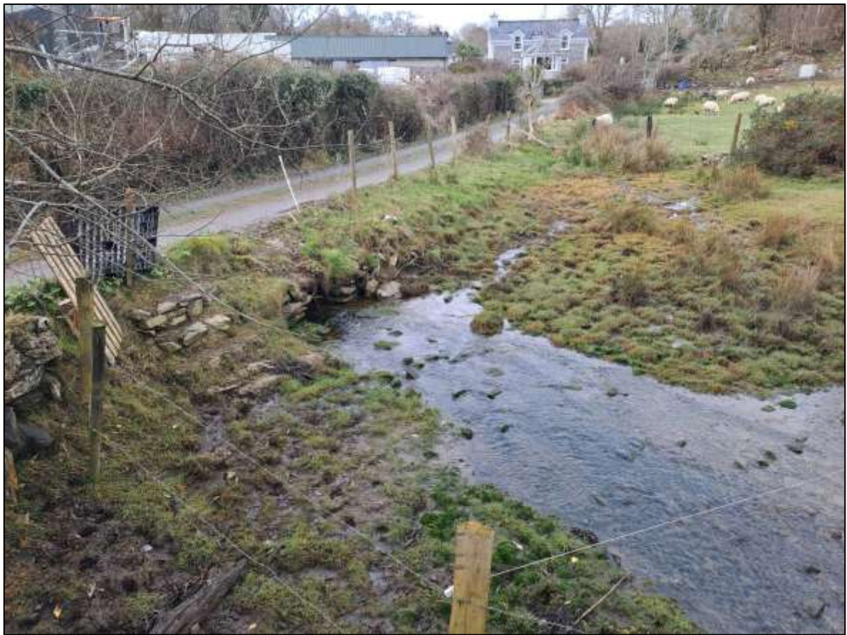
Outlet from Tubbrid Spring on east side of L7556 Tubbrid road.
