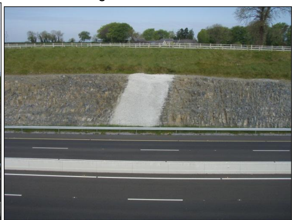
Concrete patch reinforcing weak ground.
