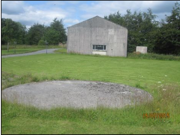
The former hoist house with the capped shaft in the foreground.
