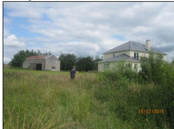
A new dwelling house is built in the centre of the site close to the shaft.
